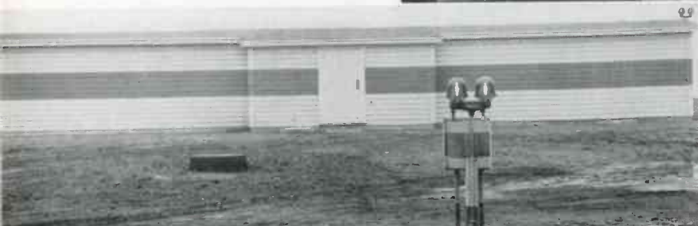
↑ "Inner marker" at LaGuardia airfield, located at start of landing runway. Projecting its radio energy upward, this marker gives pilot a final quick instrument check
