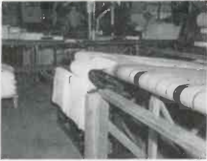
Pillow case leaving conveyor and being thrown over stacking rail
