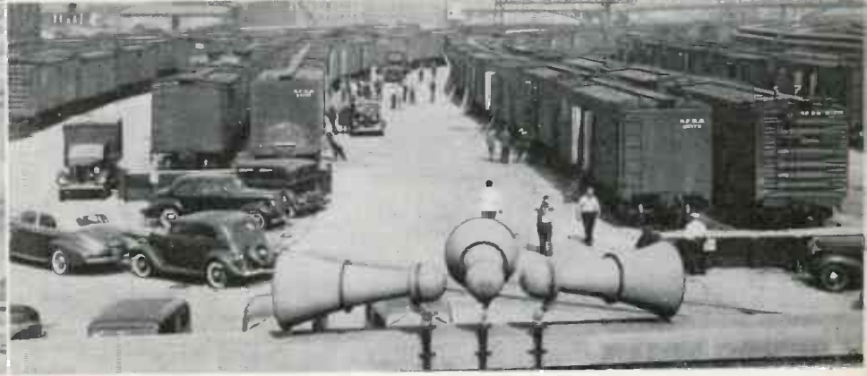
▼ Loading box-cars with war munitions is now speeded up in this Chicago freight yard by loudspeaker system covering all loading tracks
